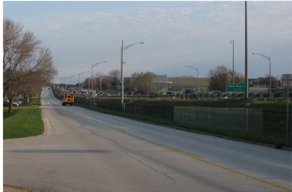
Southbound I-43 near Green Tree Rd
